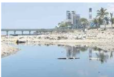
Picture #10. Contaminated Area.
